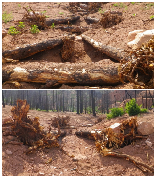
Figure 8: Log grade control structures implemented downstream of the Waldo Canyon Fire (2012), Colorado.
