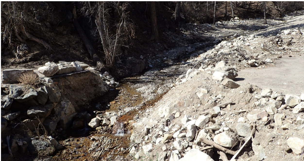
Figure 3: Wet canyon creek passing through the approaches of the (removed) historic arched culvert. Note the gravel-sized material in the streambed and the asphalt parking lot. The average channel slope upstream of AZ-366 is ~20%.
