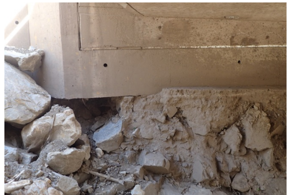
Figure 5: Erosion at the north abutment of the AZ-366 bridge over Wet Canyon.
