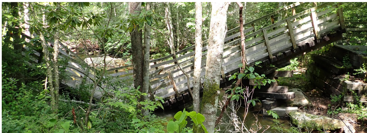
Figure 2: Failure of Virginia Creeper Trail Bridge 41 over Green Cove Creek from Hurricane Helene.
