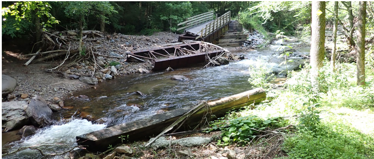
Figure 1: Failure of Virginia Creeper Trail Bridge 37 over Whitetop Laurel Creek from Hurricane Helene.
