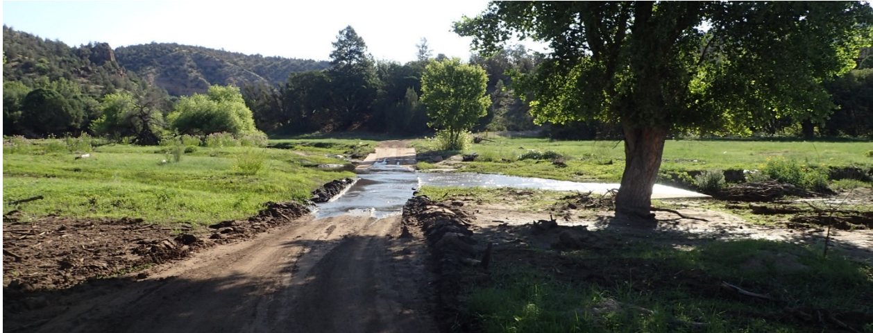
Figure 2: National Forest System Road 233 crossing of the Tularosa River (flowing left to right), with concrete crossing, downstream concrete apron, and upstream wetlands.
