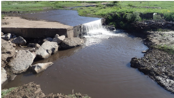
Figure 5: Scour at downstream limit of concrete apron. This is an aquatic organism passage barrier for the target species (loach minnow).
