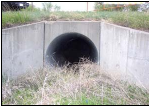
Figure 17: US-34 culvert, 6' inlet.
