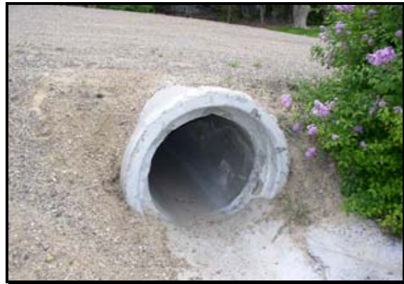
Figure 18: US-34 culvert, 2.5' outlet.
