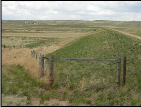
Figure 2: Upstream face of B-4 embankment. Slope = 3.5:1
