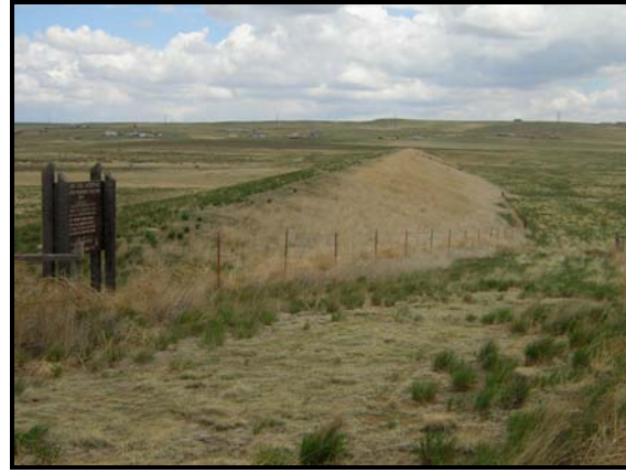
Figure 3: Downstream face of B-4 embankment. Slope = 3:1.
