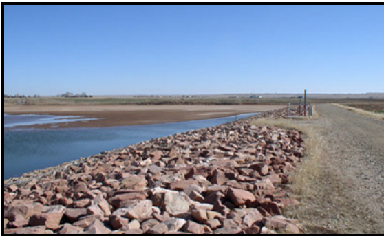
Figure 6: Upstream face of Clark Reservoir embankment.
