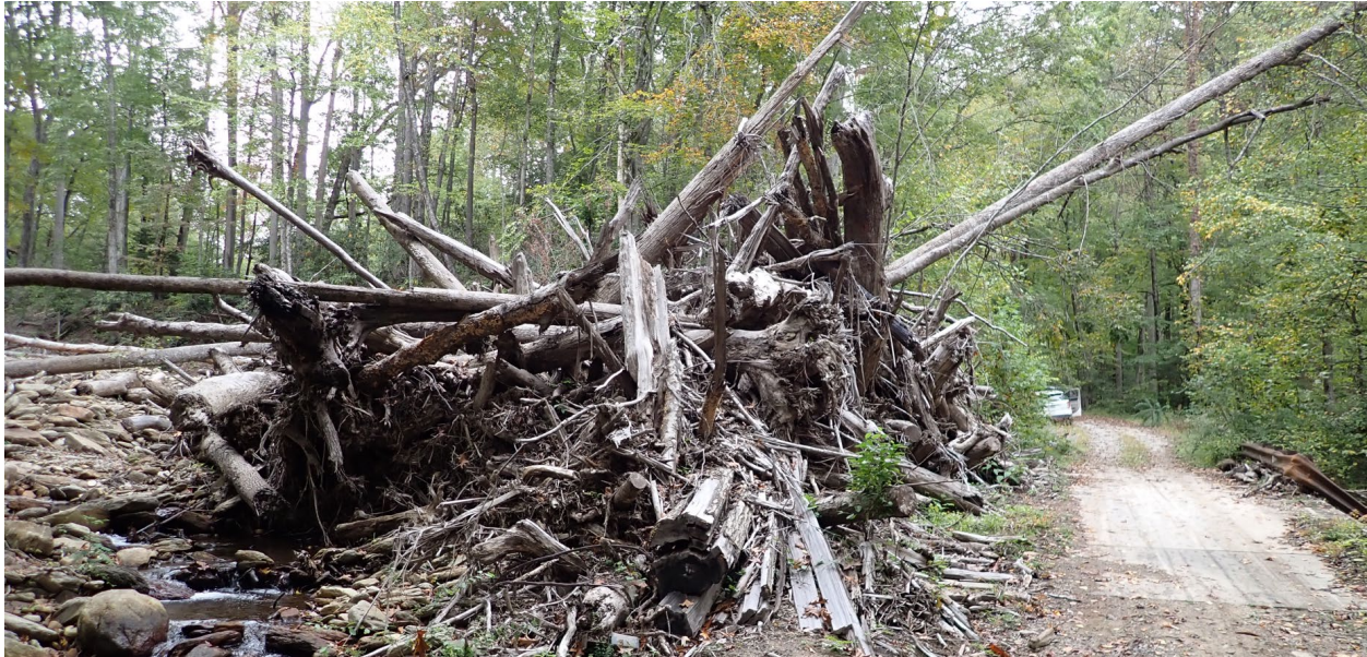
Figure 3: Large wood and rock material accumulation on a blocked bridge opening in the Curtis Creek watershed.
