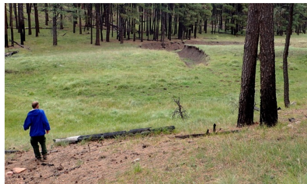
Figure 11: Dick Hart Draw, with eroded berms.
