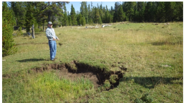
Figure 15: Active headcutting downstream of a roadway culvert.
