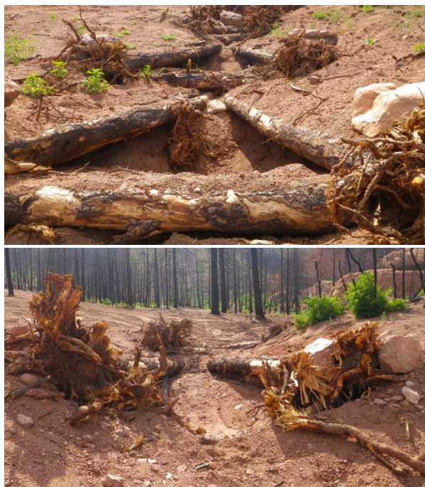
Figure 20: Log grade control structures implemented downstream of the Waldo Canyon Fire (2012), Colorado.
