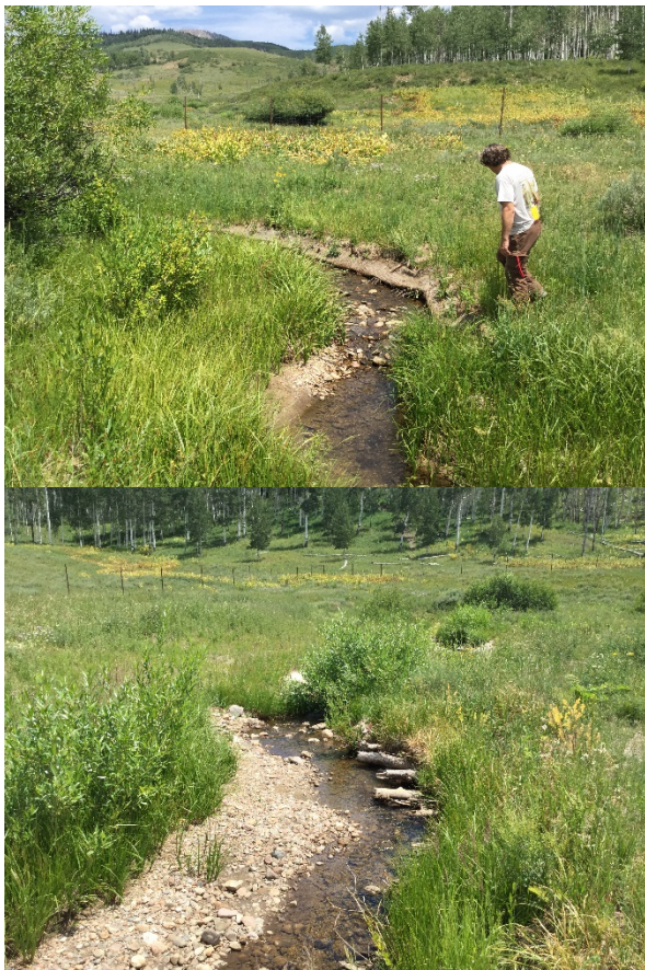
Figure 8: Undercut coir matting and toe wood armored banks on the upper restored reach of upper Armstrong Creek.
