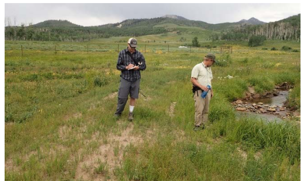
Figure 9: Earthen berm, with new channel (right) and adjacent ponds and floodplain (left).
