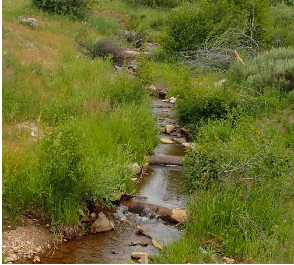
Figure 7: Rock and roll structures on upper Armstrong Creek.
