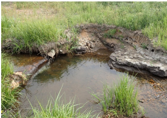
Figure 14: Erosion at downstream end of rock and roll structure.
