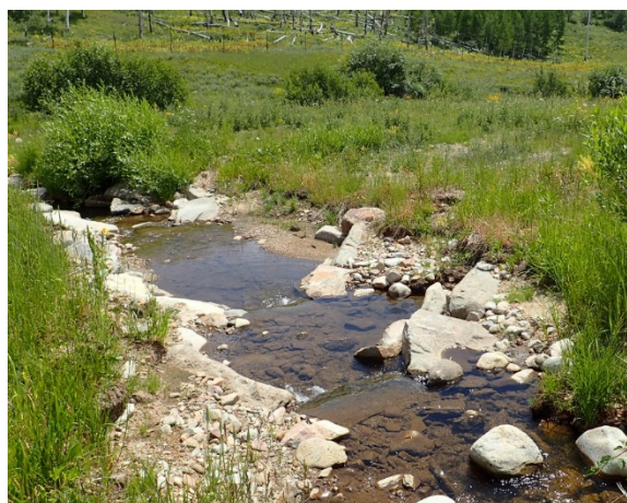
Figure 6: Rock cross vanes on upper Armstrong Creek.
