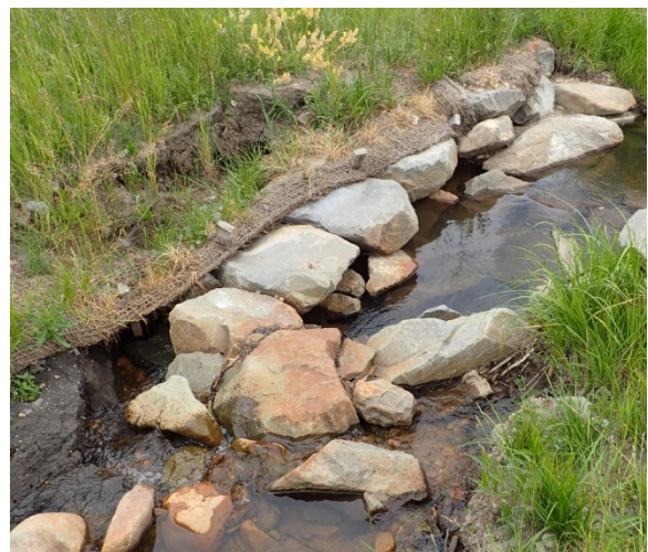
Figure 12: Piping through left arm of cross vane, with adjacent bank failure.
