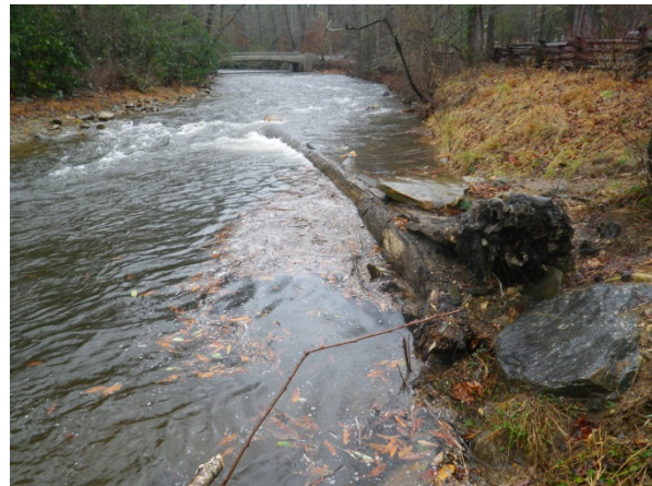
Figure 58: Log J-hook vane providing bank stabilization and pool scour 4 years after construction (Pisgah National Forest, North Carolina; photo credit: Brady Dodd).
