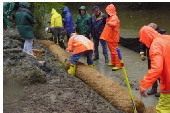
Figure 61: Installation of coir fascines (NRCS 2007, TS14I).
