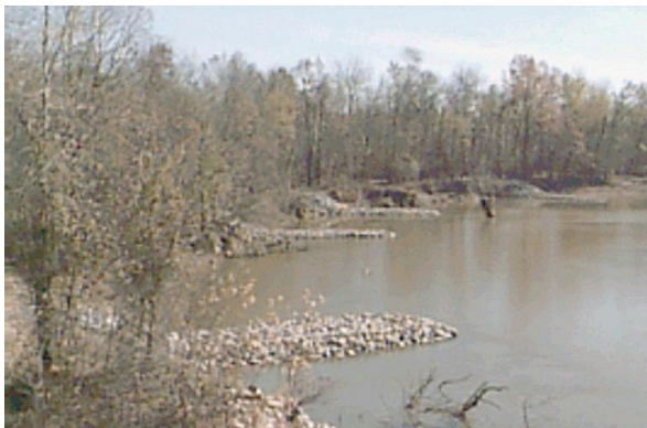
Figure 59: Bendway weir (Lagasse et al. 2009).
