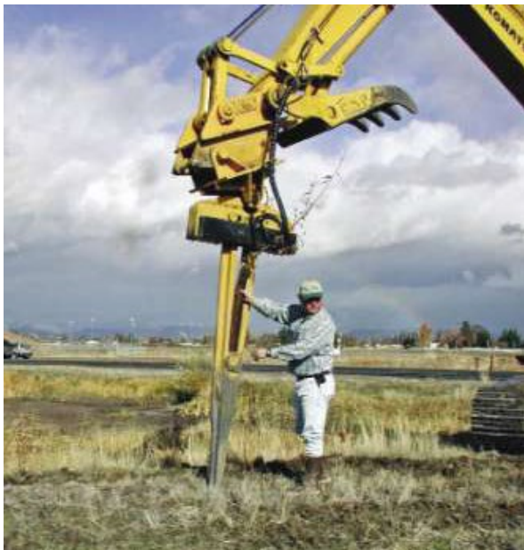
Figure 36: The use of a stinger for vegetative plantings (nativerevegetation.org).
