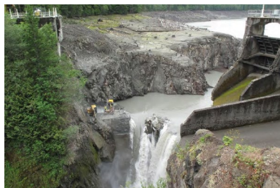
Figure 73: Removal of the lower portion of Glines Canyon Dam, Washington, 7/1/2012 (photo courtesy of the National Park Service).
