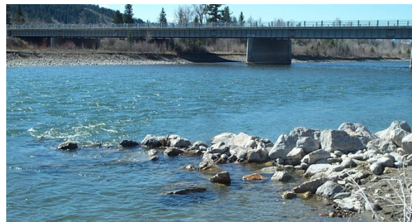
Figure 55: Stream barb (courtesy Jon Fripp).
