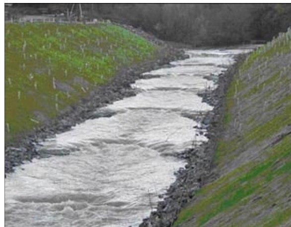
Figure 50: Pool and weir fishway.
