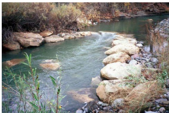
Figure 67: Cross vane on the Rio Blanco, CO (NRCS 2007, Ch11).
