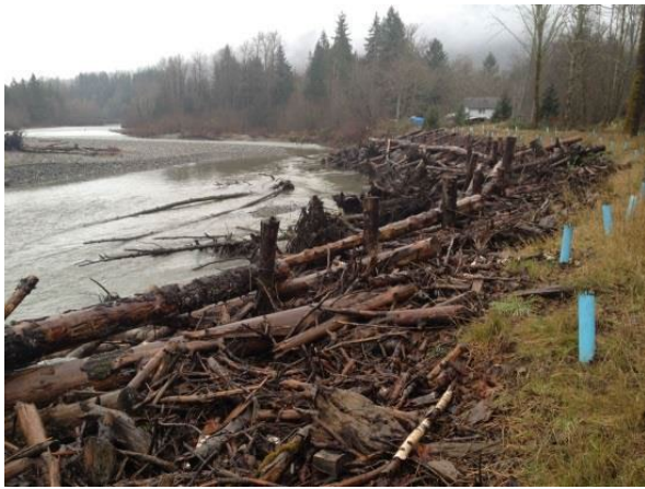
Figure 44: Complex timber revetment (photo credit: Tim Abbe, USBR and ERDC 2016).
