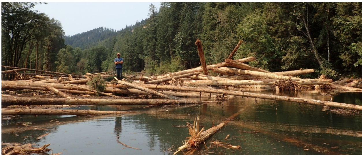
Figure 25: Stage 0 restoration on the South Fork McKenzie River, just after phase 1 construction (8/7/2018).
