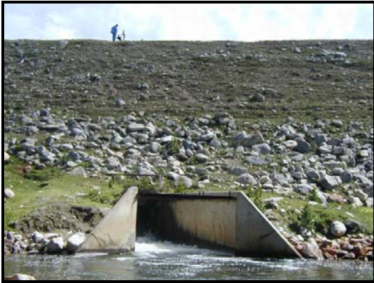
Figure 3: Principal spillway outflow.
