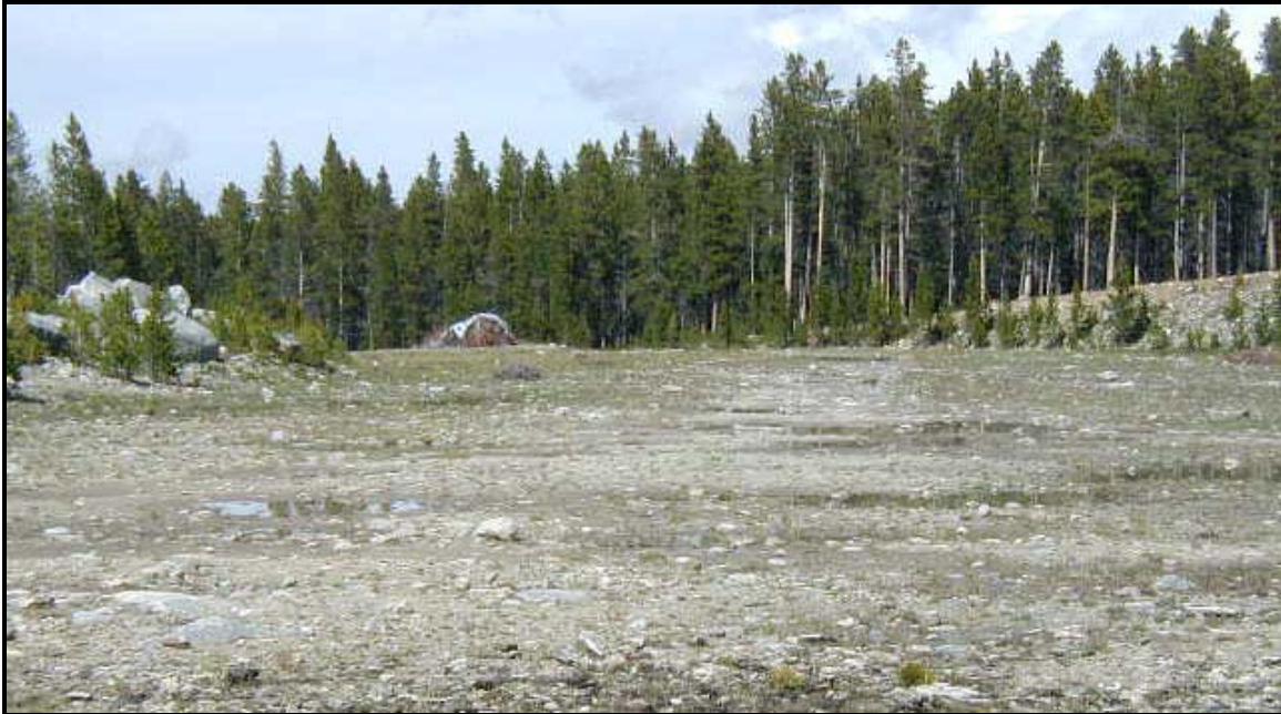
Figure 14: Emergency Spillway, Willow Park Reservoir. Capacity \approx 8100 cfs.
