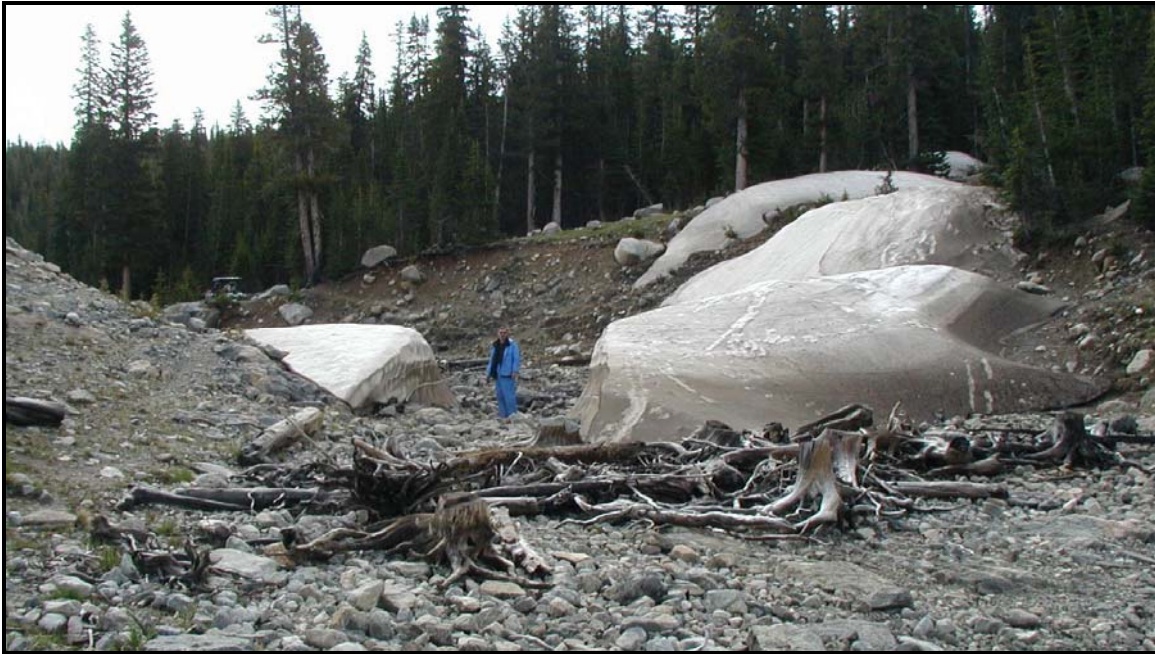
Figure 11: Emergency Spillway, Cloud Peak Reservoir. Capacity \approx 1900 cfs.
