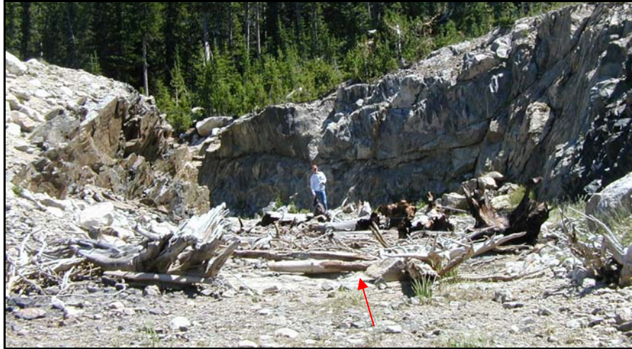
Figure 2: Emergency spillway entrance, facing downstream. Flow capacity is approximately 1800 cfs with water-surface-elevation at the dam crest.
