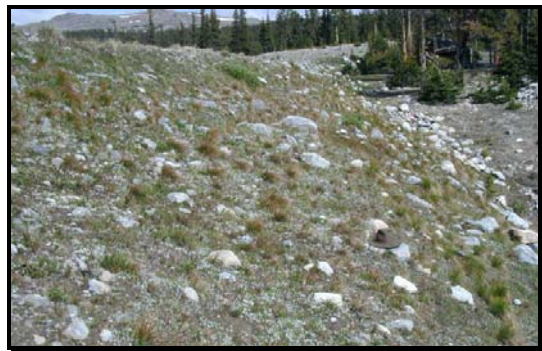
Figure 4: Downstream embankment face, Cloud Peak Reservoir.
